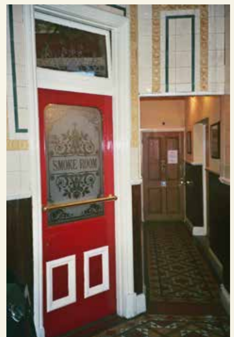
The side passage at the Woodman, showing the Minton floor tiles, and the smoke room door, as well as the wall tiles.
