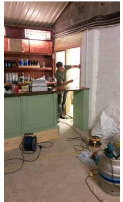
Building work in progress for the brewery bar and shop
