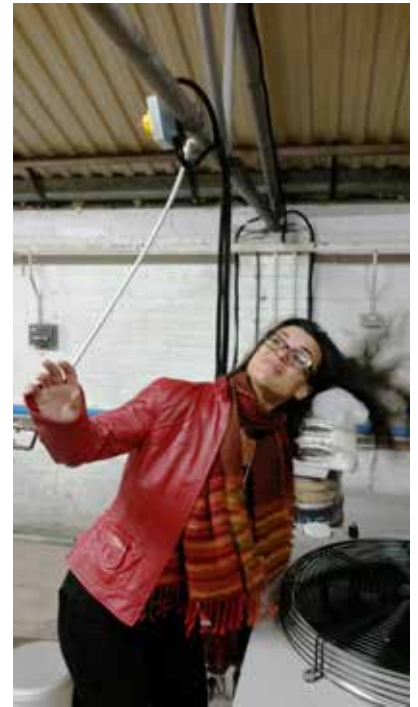
Dawkins shareholder Jane Dutson tests the cooling fan in the new brewery
