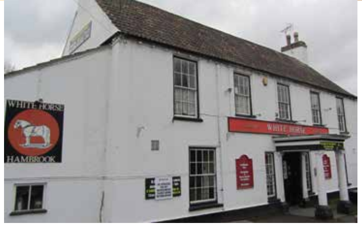
The White Horse at Hambrook undergoing refurbishment
