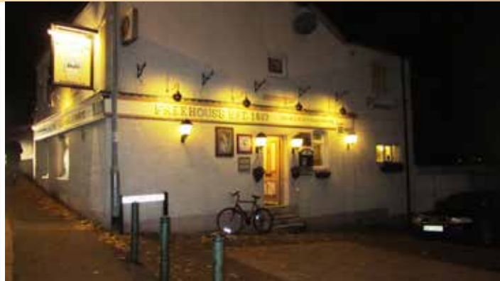
The split-level Borough Arms is perched on the edge of the bridge over the West Coast Main Line railway
