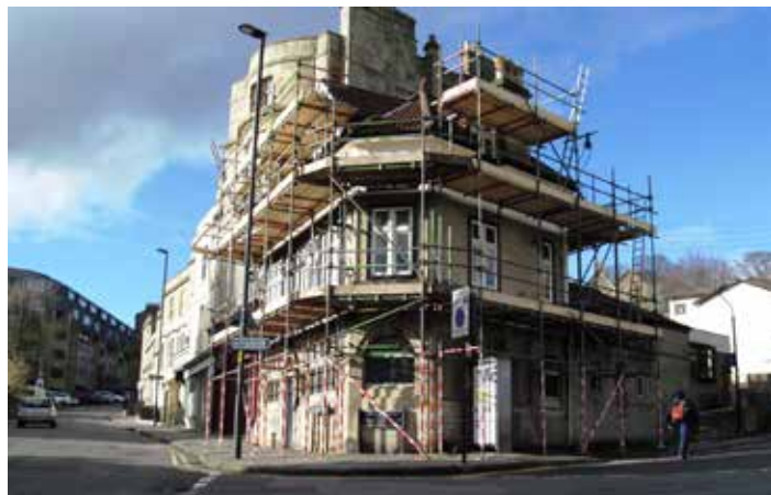
Ye Olde Farmhouse surrounded by scaffolding
